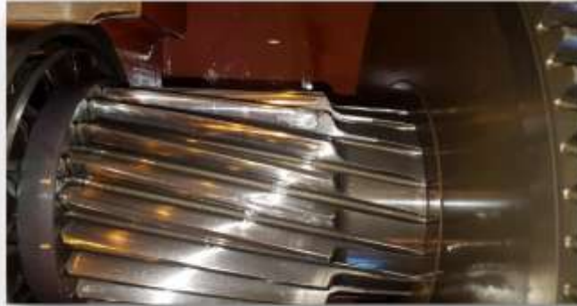
Damaged gearing and bearings
